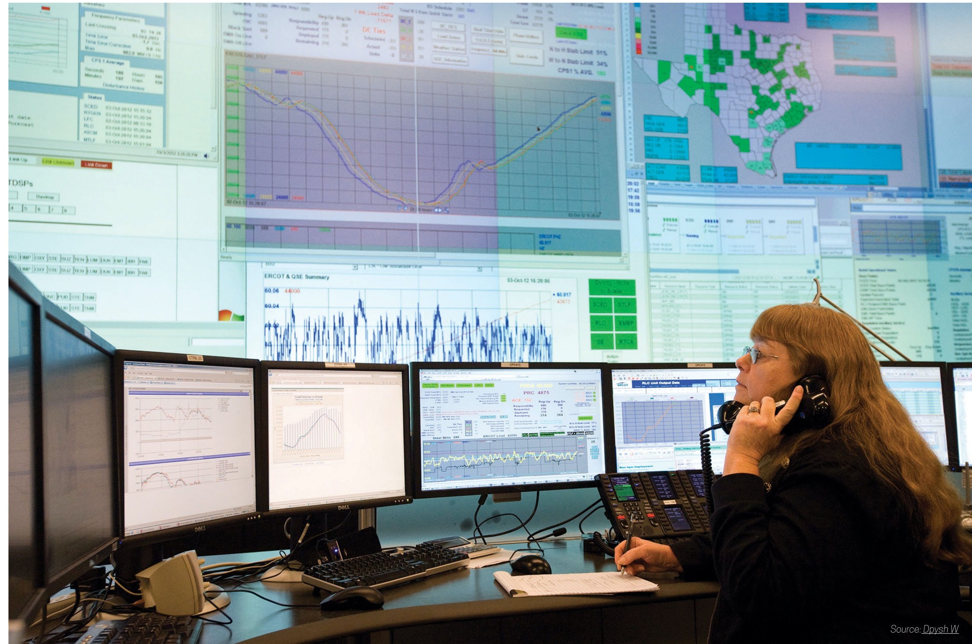
ERCOT Grid Control center in Texas
